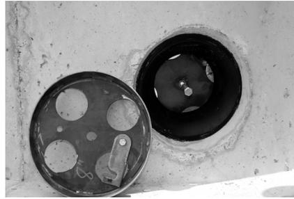
3. Lightly tap the alignment post on the core half of the mandrel three to five times. The vibration of this action will loosen the mandrel half from the concrete.
