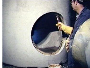
Pipe-end O.D. should be lubricated to a length 6” longer than the insertion length. **(With connectors rated for standard service, hydrocarbon-based lubricants must NOT be used, as these have a detrimental effect on the connector material and its watertightness rating.)**
