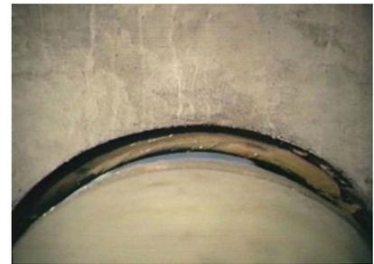
6. Insert pipe into connector to an insertion length sufficient to ensure that pipe wall is in touch with gasket around the complete circumference, and a minimum length of 6” (subject to benching dimensions) protrudes beyond the gasket sealing surface. Pipe must always be inserted “straight”. Any required deflection should be applied after pipe has been inserted into connector.
